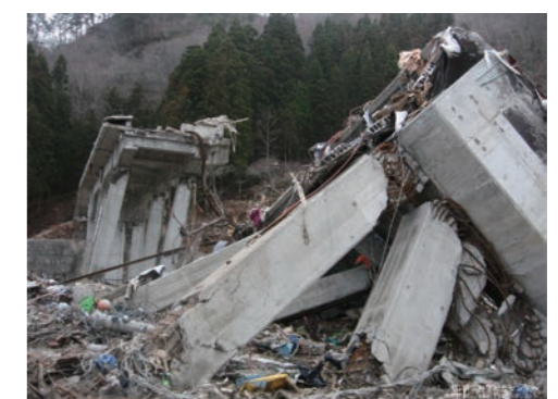
Shimanokoshi Station in ruins Source: Institute for Fire Safety and Disaster Preparedness
