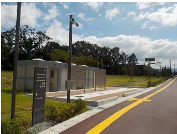
Photo8 : Park restroom with a security camera
