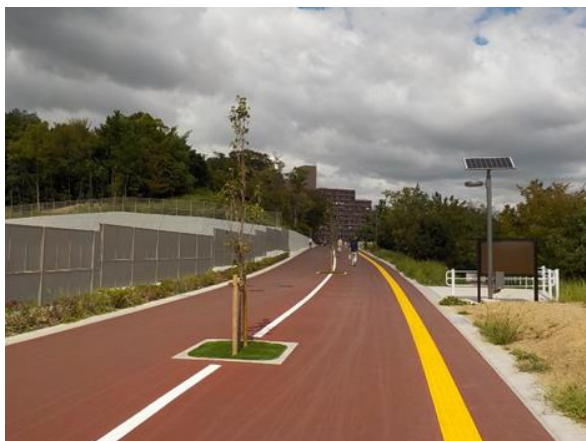
Photo9 : Park road built with consideration for user safety
