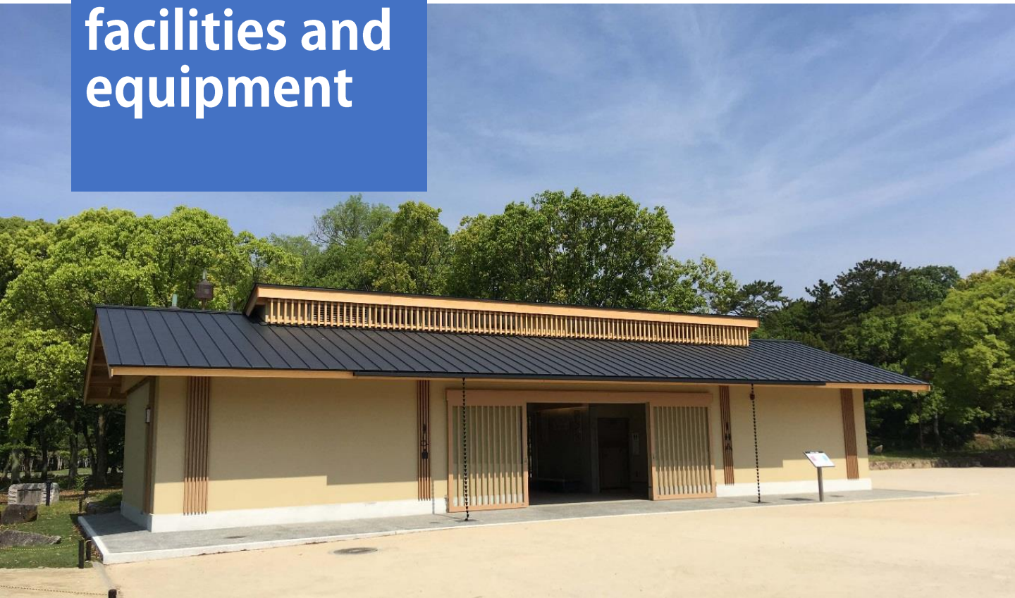
Photo5: Omotenashi [hospitality] Restroom installed in Daisen Park
