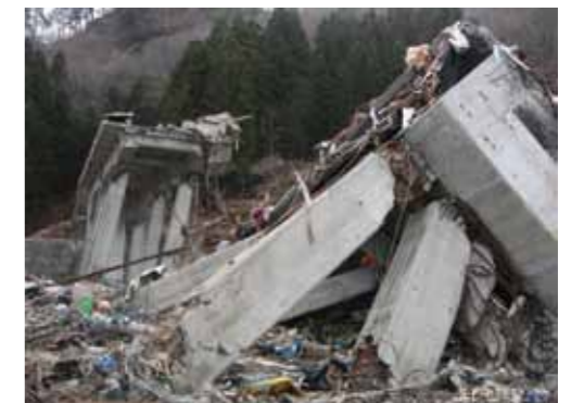
Shimanokoshi Station in ruins Source: Institute for Fire Safety and Disaster Preparedness
